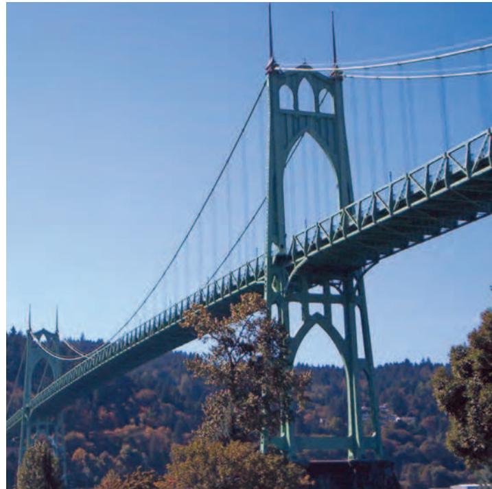
St. John's Bridge Portland, OR Photo courtesy of National Bridge Alliance
