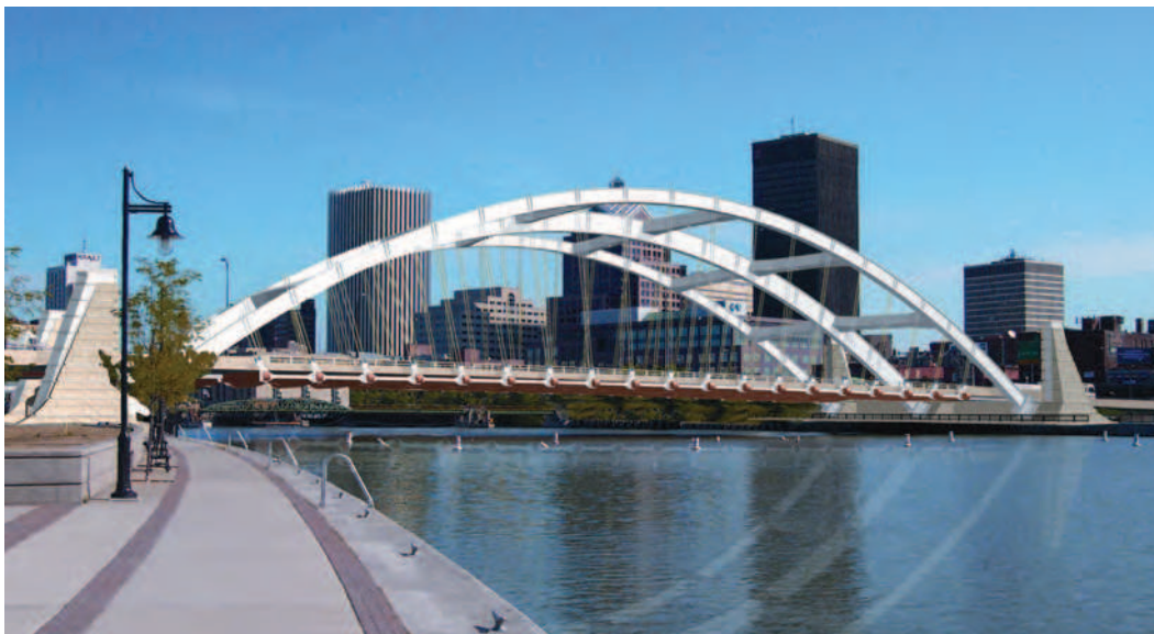
Troup-Howell Bridge Rochester, NY
